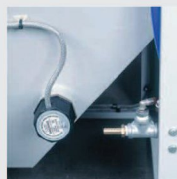
Electric Sump Heater Element
